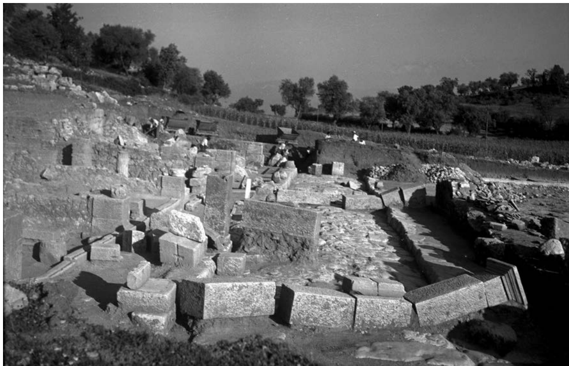
Fig. 2 – Alba Fucens: pillars collapsed across Via dei Pilastrì. Due to the collapse, the operation of the road ceased until the modern archaeological excavation and the subsequent restoration of the pillars (courtesy of Soprintendenza per i Beni Archeologici dell’Abruzzo).
