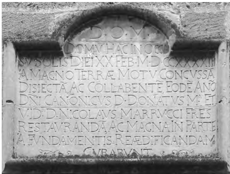
Fig. 8 - Memorial stone recording the damage (... a magno terraemotu concussa ...; struck by a great earthquake) in the Marruci Palace (Francavilla Fontana) in the 1743 earthquake.
