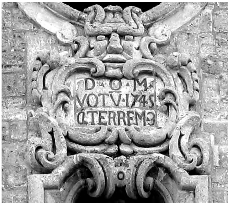
Fig. 5 - Nardò: memorial stone recording the collapse of the San Domenico bell tower.
