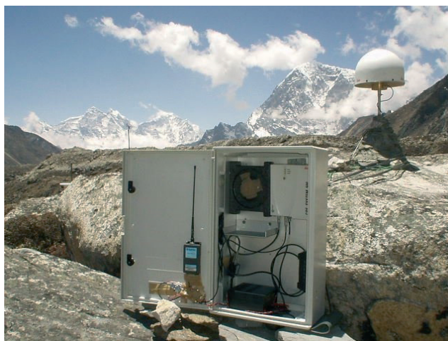
Fig. 2 - The equipment of the Leica 530 station with choke ring antenna.
