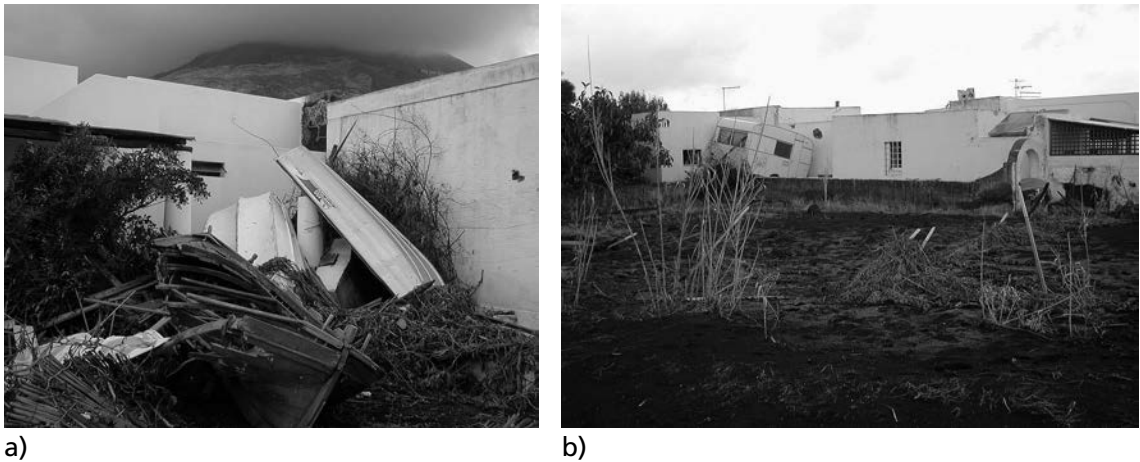
Fig. 4 - Tsunami damage observed at Scari. Both images were collected on January 13, 2003: a) boats carried onshore and thrown against house walls, uprooted vegetation and damaged buildings were typical tsunami signatures observed at Scari; b) a caravan moved away from its original location and a bent fence.
