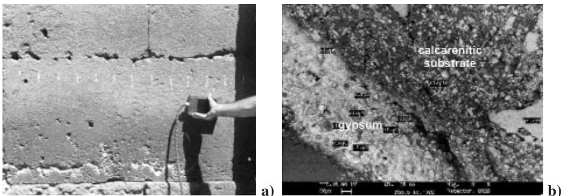
**Fig. 2** - Patinas at the Ucciardone wall: a) patina is much more noticeable in the lower half of the block. Notice transition of the process of patina growth. b) SEM microphotograph of patina. This primarily comprehends gypsum and, subordinately, calcium oxalate dihydrate. Black marks refer to EDS analysis here not reported. Notice the interface between the calcarenitic substrate and gypsum.
