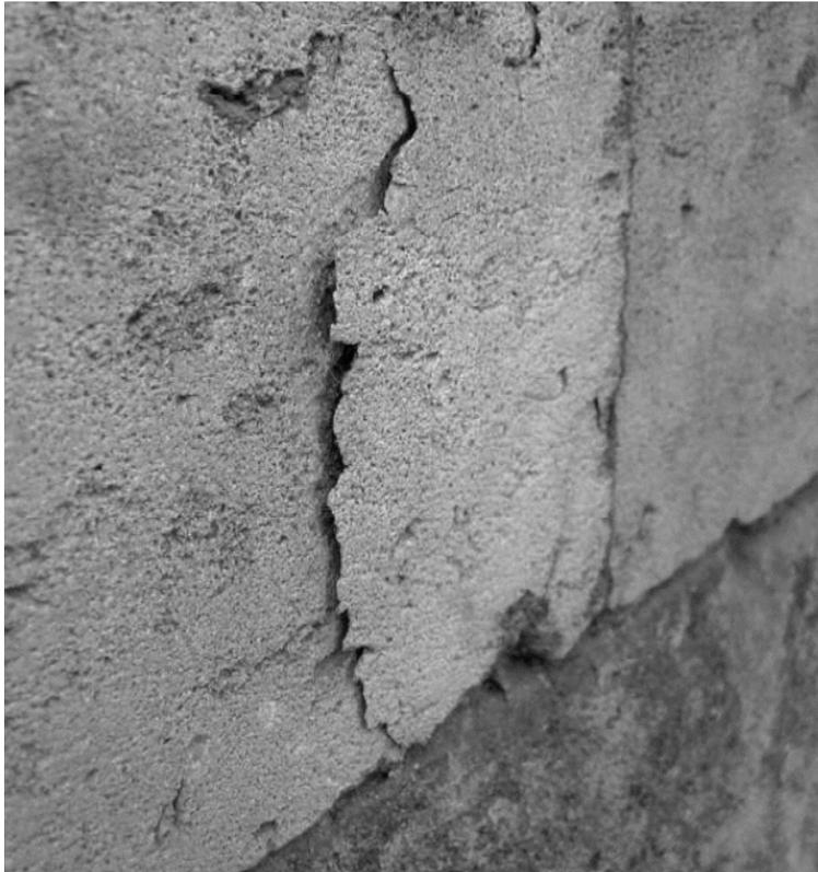
**Fig. 7** - Example of process of advanced patina exfoliation at site B. Here the patina is composed mainly of gypsum.
