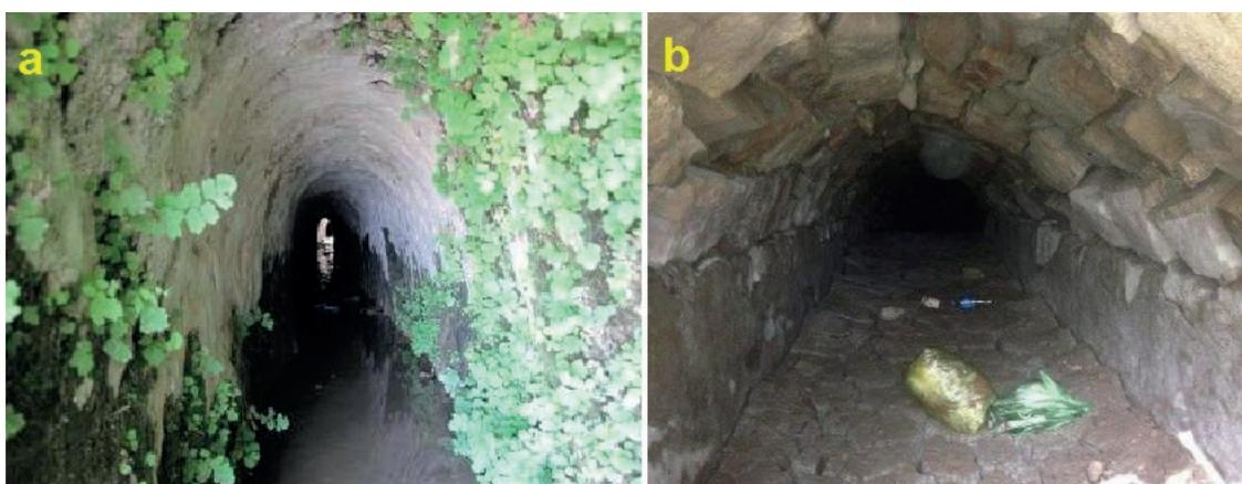
Fig. 2 - Photographs showing examples of *karez*es design in Iraq: a) round arch *karez* tunnel in limestone at Zimzimuk (Lightfoot, 2009), b) *karez* tunnel in limestone at Sulaimaniyah city (Al-Manmi et al., 2019).
