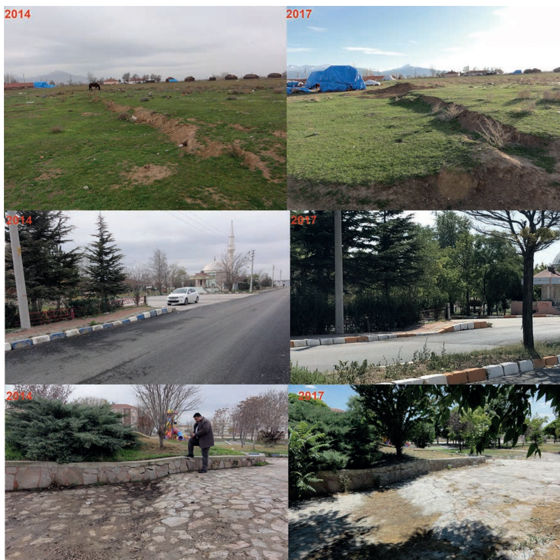
Fig. 2 - Field photographs showing the vertical displacement along surface deformation.
