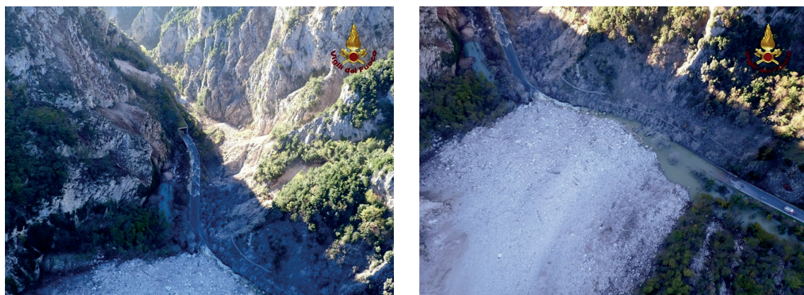
Fig. 3 - The rockfall triggered by the 30 October 2016 earthquake on the SP 209 and Nera River ( https://www.perugiaday.it/foto/cronaca/terremoto-norcia-frane-valnerina/aa644aa1.html#&gid=1&pid=1 ).
