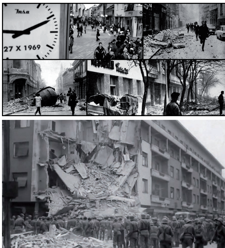
Fig. 1 - Damage in Banja Luka caused by the 1969 earthquake.
