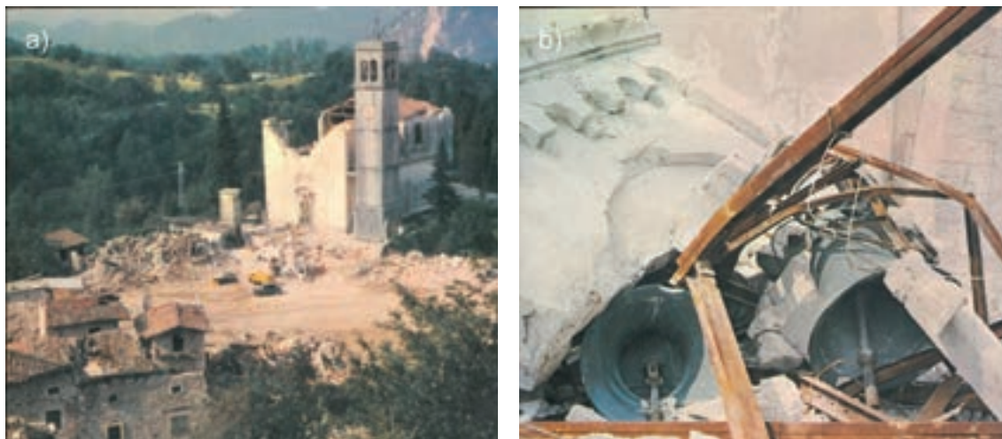
Fig. 1 - Typical damage observed in the epicentral region of the Friuli earthquakes [after CNEN-ENEL (1976): photos by Diego Molin]. The left photo shows a view over parts of Forgaria del Friuli [pers. communication by Dario Slejko].
