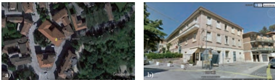
Fig. 10 - E. Ricciardi elementary school building: a) plan view of the school; b) external view of the building where the connectors installed after the 1997 central Italy earthquake are visible.
