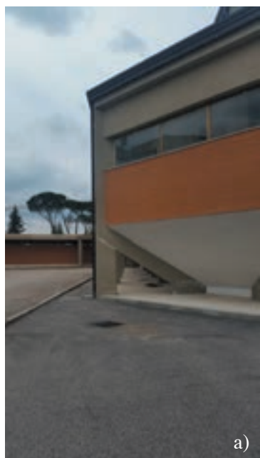
Fig. 9 - Ciancarelli high school building: a) RC columns of the gymnasium originally designed (end of 1970s) as short-span oblique cantilevers and modified by the addition of the vertical lower column during recent (2014-2015) seismic retrofitting; b) small cracks at the structural joint.
