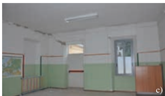
Fig. 17 - B. Tucci primary school building: a) plan view of the school complex; b) shear crack in vertical load-bearing elements; c) cracks between floor and masonry bearing walls.
