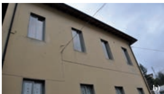
Fig. 17 - B. Tucci primary school building: a) plan view of the school complex; b) shear crack in vertical load-bearing elements; c) cracks between floor and masonry bearing walls.
