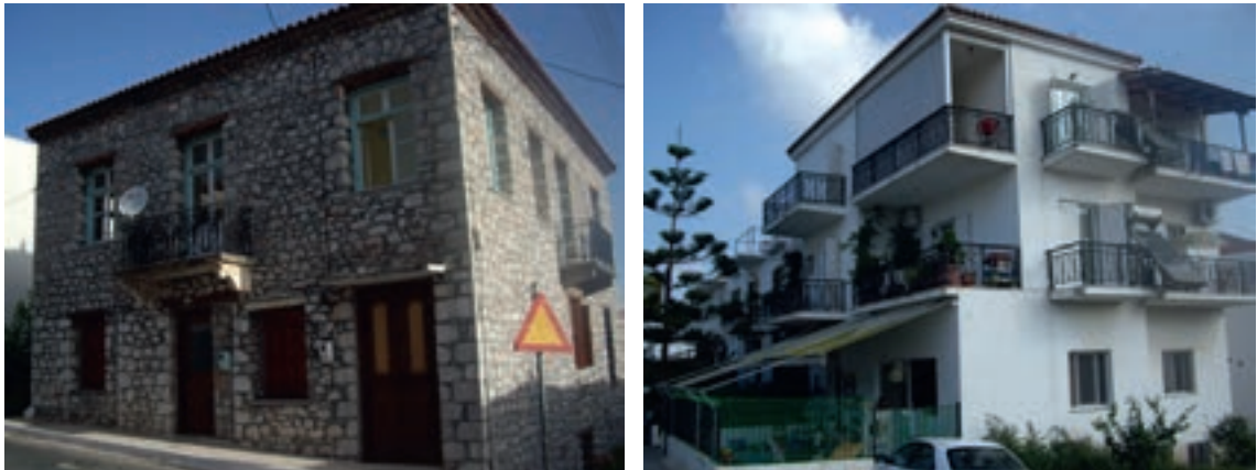
Fig. 3 - A typical two-storey residential unreinforced load-bearing stone masonry building (left), a typical 3-storey RC frame with infill masonry walls apartment building of the period 1985-1994 (right).
