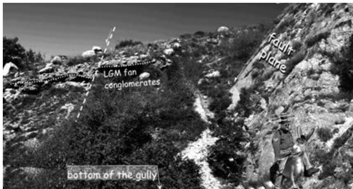
Fig. 9 - Photograph of view looking W of the Late Pleistocene faulted conglomerates (dashed line, one of the splays) at the apex of a fan crossing the Magnola fault. Note on the right the main fault plane exhumed by the deep, recent gully erosion (area of Forme village; PM piggyback of Donkey included for scale; photograph by PG).
