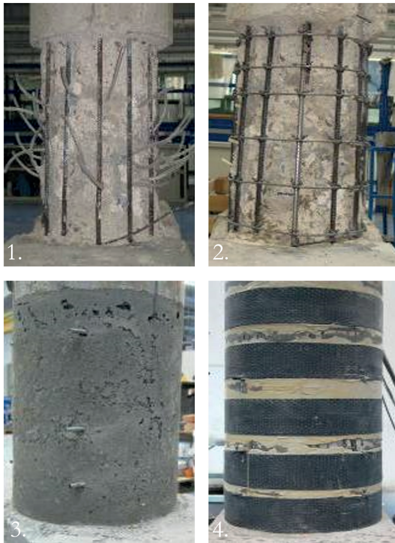
Fig. 7 - Experimental samples of CFRP application onto a concrete column, in the following order: 1) removal of damaged concrete and epoxy resin injections; 2) replacement of the bars; 3) restoration of the concrete surface; 4) application of transverse and longitudinal CFRP jacketing.
