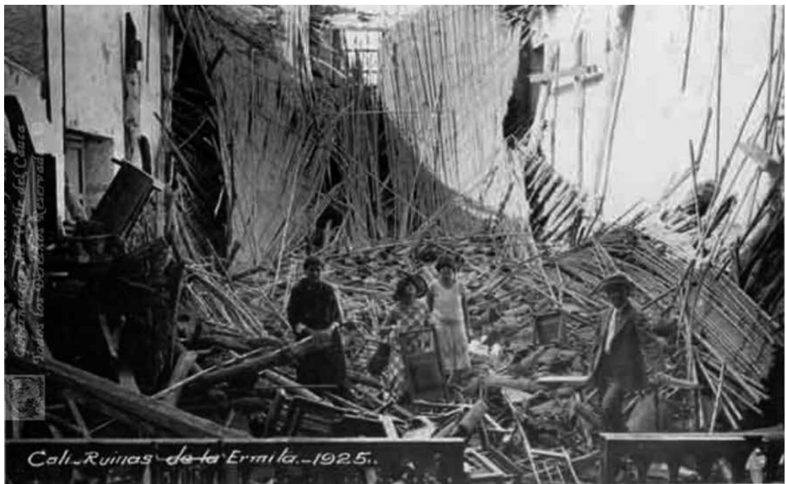
Fig. 3 - The ruins of the church 'Ermita Vieja de Cali', in Cali, totally destroyed by the 7 June 1925 earthquake (Barth, 1925; Calero Tejada, 1983).
