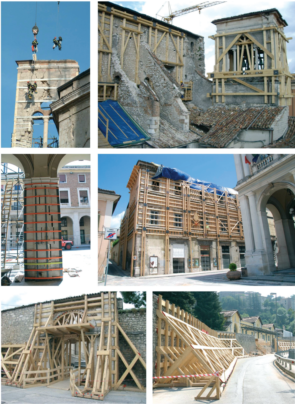
Fig. 7 - Examples of provisional works realized by the Italian National Fire Department in the L'Aquila area.
