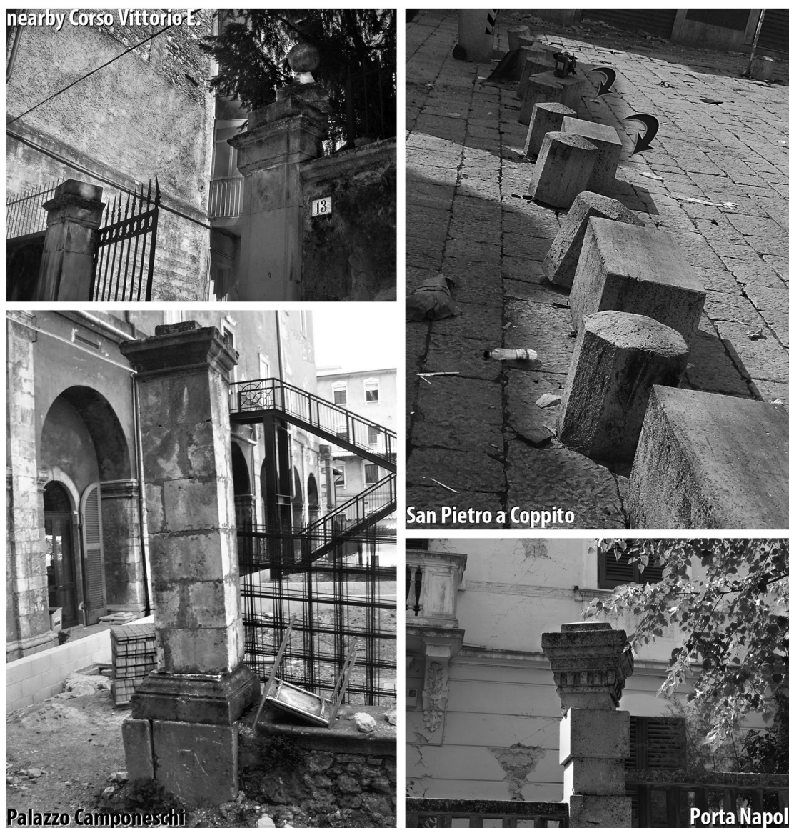
Fig. 5 - Examples of ffd rotations observed in downtown L'Aquila.
