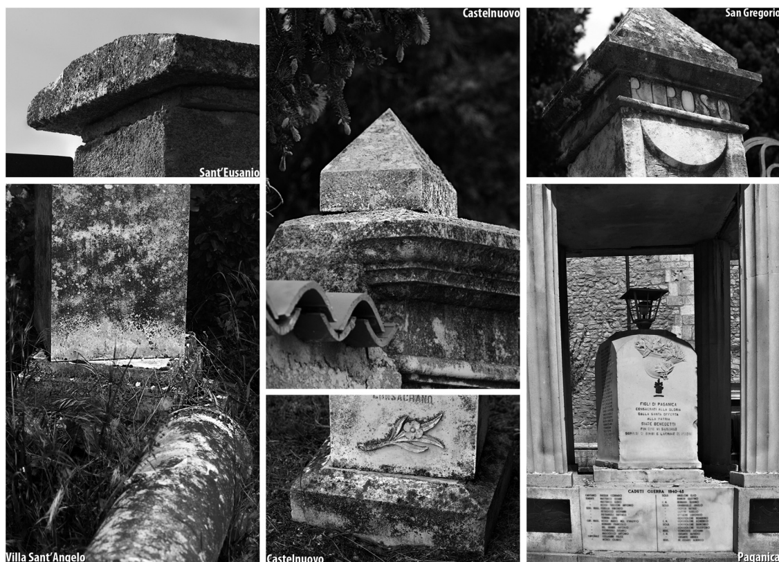
Fig. 3 - Examples of ffd rotations observed following the L'Aquila earthquake.
