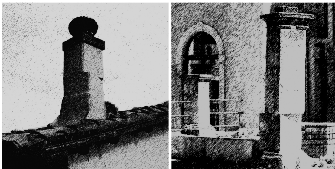
Fig. 2 - The sketch represents the two main typologies of rotations observable in the field: a) building-based object: chimney in Pianola (3 km from the epicentre), building-based objects like chimneys, furniture and some pillars are usually placed on top of a building or a construction and can be affected by rotational modes of the underlying structure; b) free-field object: pillar at the L'Aquila University (2 km from the epicentre), free-field objects like tombstones, gate pillars, capitals, monuments and some statues rest directly on the ground, are considered reliably representative of pure rotational ground motion, and constitute the data set of this work.
