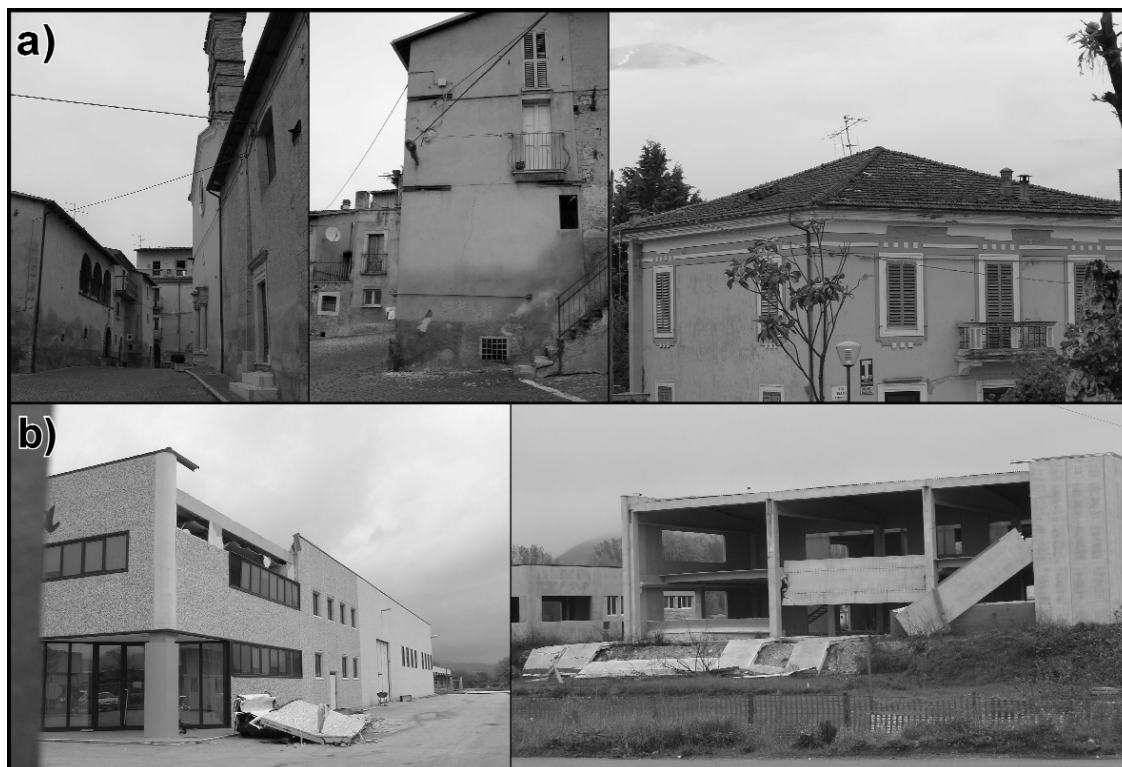
Fig. 6 - Monticchio, examples of damaged buildings with different vulnerability: a) historical centre, class B, slight damage (grades 1 and 2) (photo a, on the right by I. Cecic); b) industrial district, classes D-E, moderate damage (grade 3) (photo b, on the left by M. Godec).
