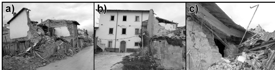
Fig. 2 - Examples of variation of the vulnerability class associated to masonry buildings: a) class B house with external intervention, but the collapse reveals a wall structure typical of vulnerability class A; b) class B edifice (in the background) where the reinforcing prevented significant damage, so the effective vulnerability class becomes C (photo by A. Tertulliani); c) class B house elevated and restored using different materials that create heterogeneity in the structure and overloading; the final behaviour is like a building of vulnerability class A.
