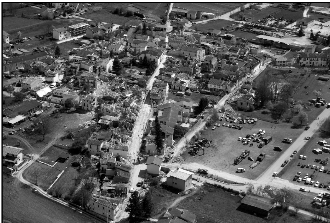
Fig. 4 - Onna (photo by A. Tertulliani): aerial view showing destruction but also standing edifices (grades 2 and 3 of damage).
