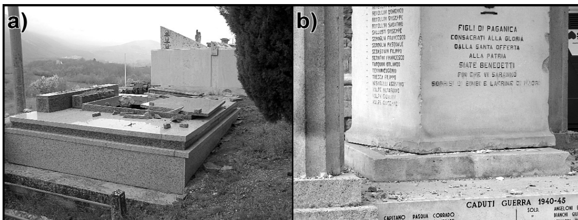
Fig. 11 - a) San Demetrio cemetery, overturned tombstone (photo by I. Cecic); b) Paganica, rotated war memorial.
